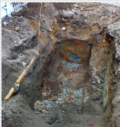
Oil/Fuel tank removal
