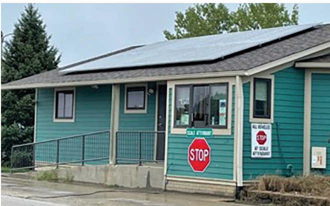
SCISWA installed rooftop solar arrays on its scale house and education center.
