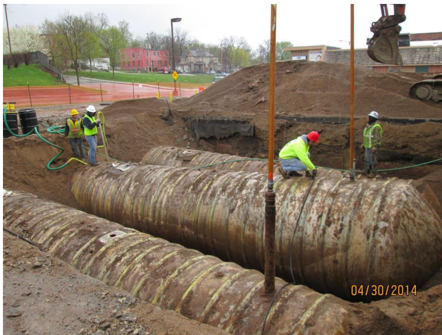
A Des Moines May 2014 tank removal of three 12000 gallon fiberglass tanks.
