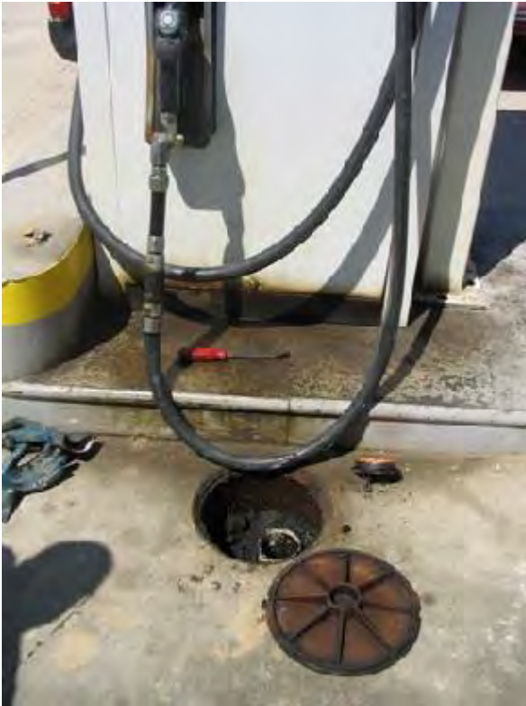
This may be a poor location for a monitoring well. Notice how the concrete around the well is not built up to avoid infiltration from surface contaminants.
