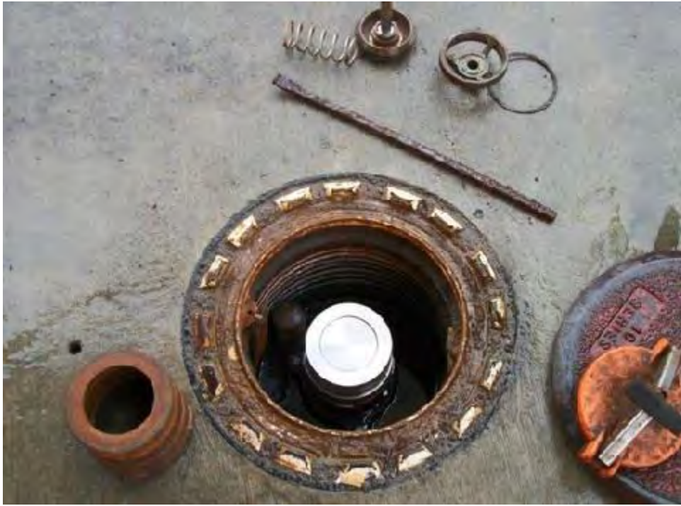
Replaced Dry Break
