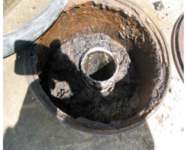
Examples of damaged monitoring wells that are at risk of being conduits for contaminants to the subsurface.
