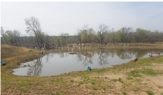
Constructed wetlands in partnership with WCSC
