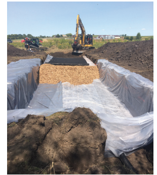
Installing a bio-reactor at MWA
