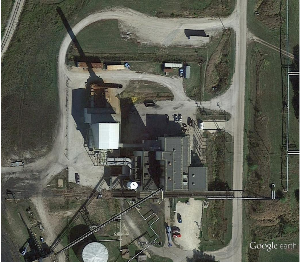
Figure 3-3 . Iowa Army Ammunition Plant boiler.
