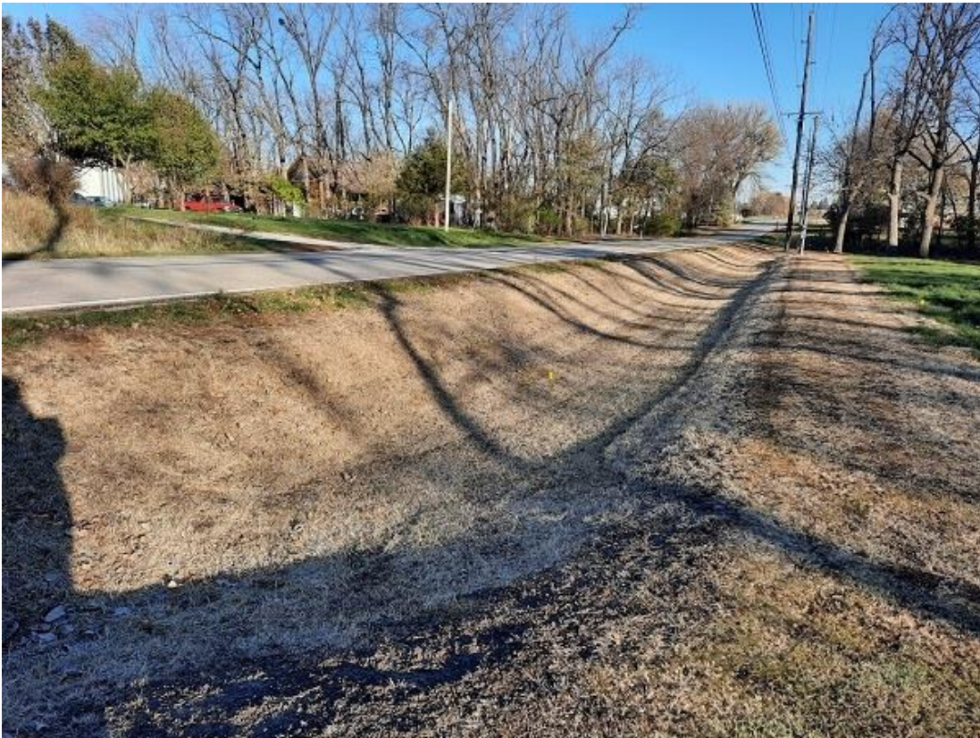
In this area, herbicide was used to kill lawn grass and other weeds in preparation of planting prairie seed.
