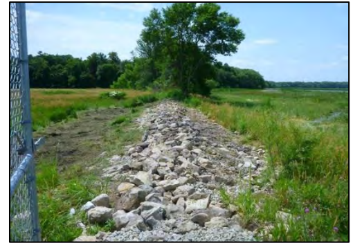
Rock fish barrier at Silver Lake
