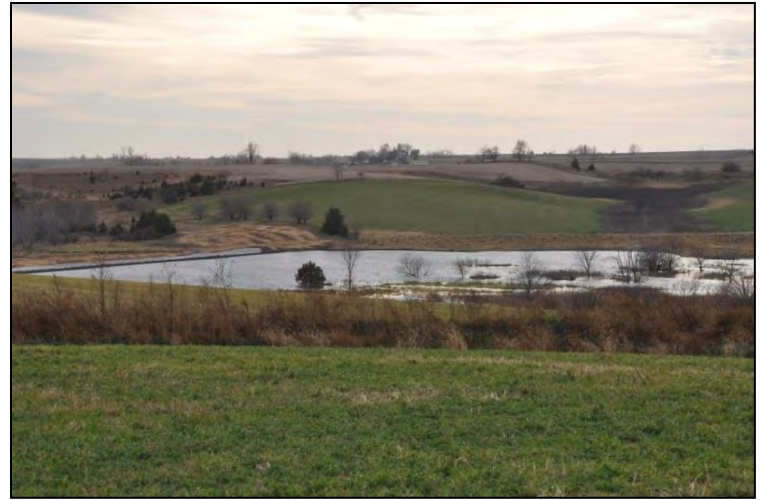
40-acre wetland structure above 12-Mile Creek Lake.
