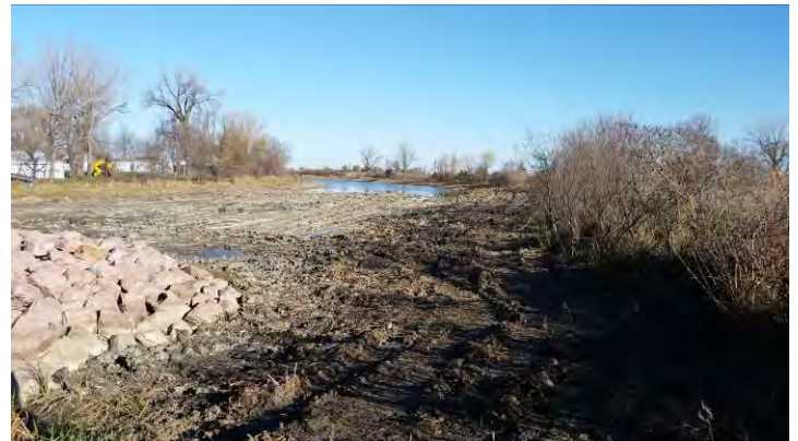
Completed construction on Nebowa Bay in Fall 2016
