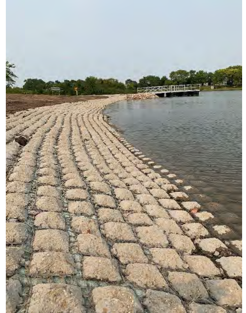
Flexamat (pictured here) was installed along the shoreline in 2020 to protect the lake from erosion and provide access to the water.
