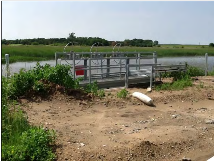
Constructed electric fish barrier in the Lost Island Lake watershed.
