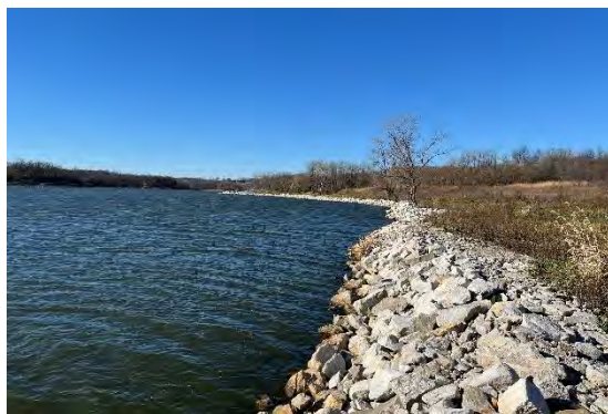
Shoreline stabilization at Rock Creek Lake (Jasper County) helps prevent erosion
