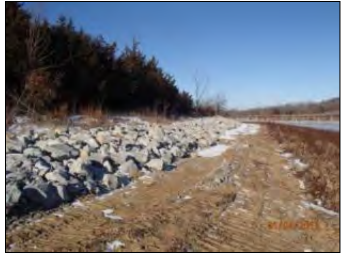
Shoreline stabilization of regions with significant erosion
