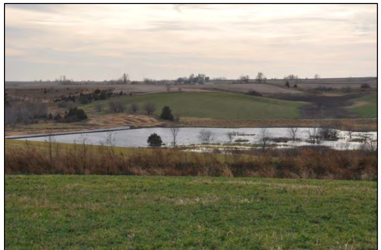
40-acre wetland structure above 12-Mile Creek Lake that protects the lake.
