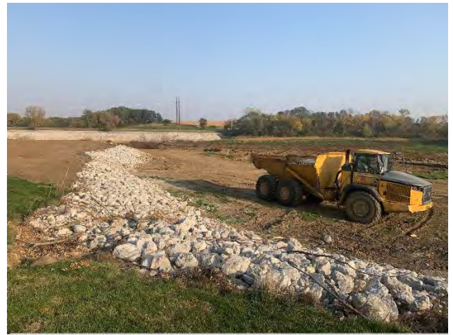
Shoreline stabilization along the banks of Lake of the Hills. Over 1000 feet of shoreline are being armored as a part of this project.
