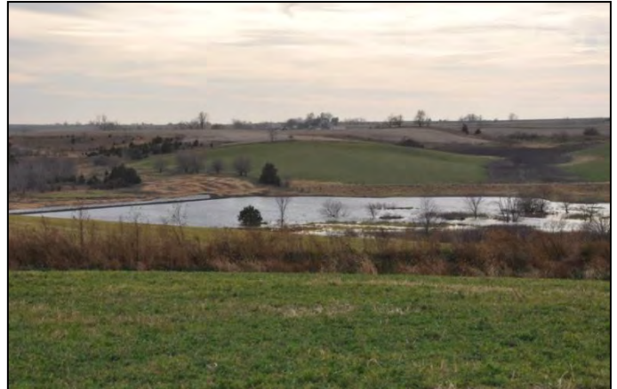
40-acre wetland structure above 12-Mile Creek Lake.
