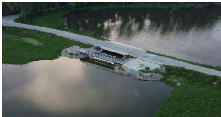
Fish barrier and pump system installed between Black Hawk Lake (top of photo) and Provost Slough (the lake's inlet)
