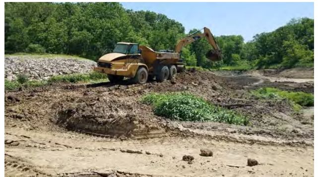
Construction equipment removes excess sediment from the lake bottom
