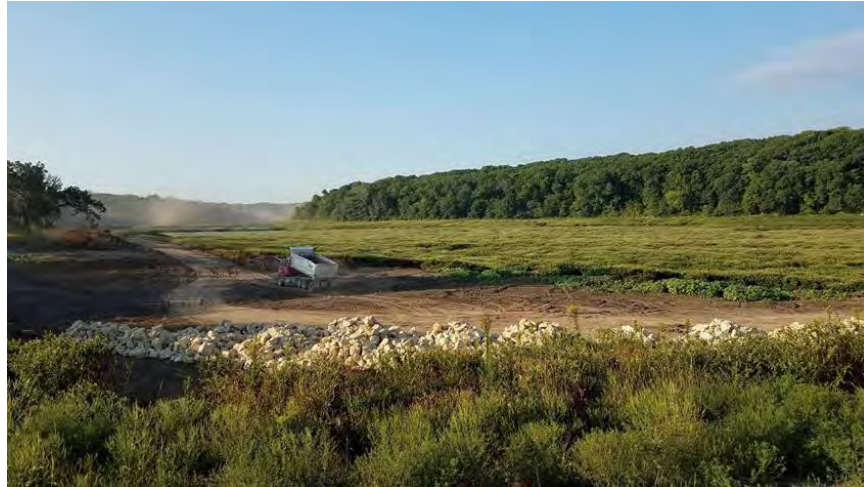
Targeted sediment removal and shoreline stabilization at Lake Ahquabi (Warren County)
