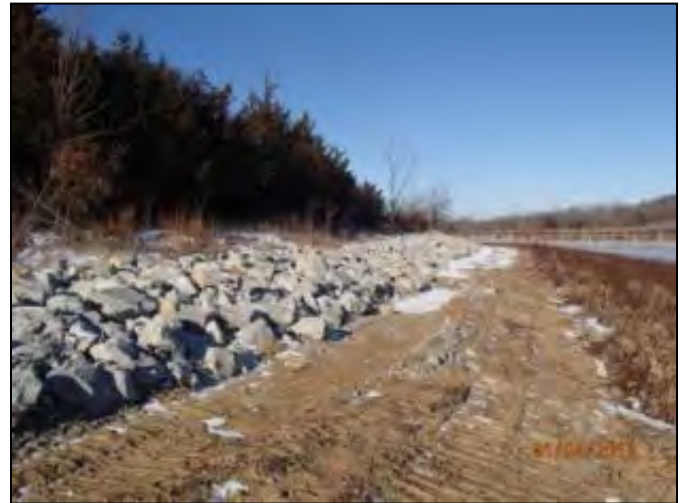
Shoreline stabilization of regions with significant erosion
