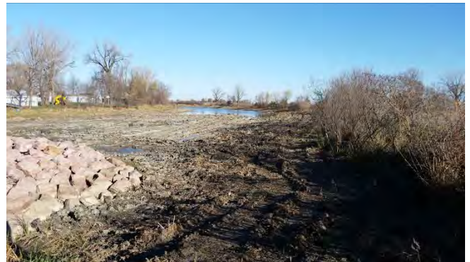
Completed construction on Nebowa Bay in Fall 2016
