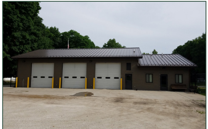
Park headquarters - separate staff entrance/work area
