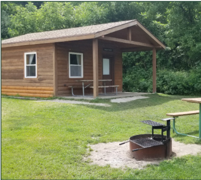
Existing Camping cabin
