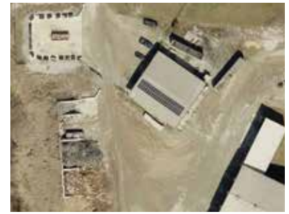
Roof-top solar array on the transfer station in Keokuk.
