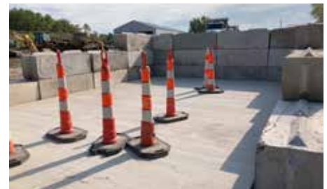
Construction of concrete bunker for glass storage at MCSWMC.
